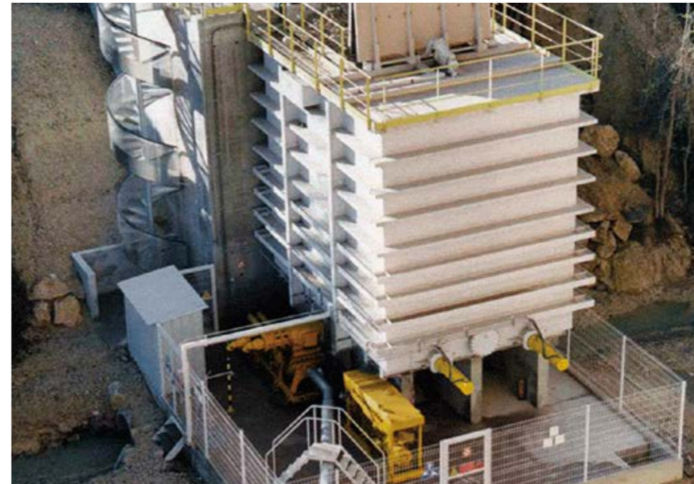
Co-incineration of alternative fuels in the cement plant of Lafarge in Le Teil, France
